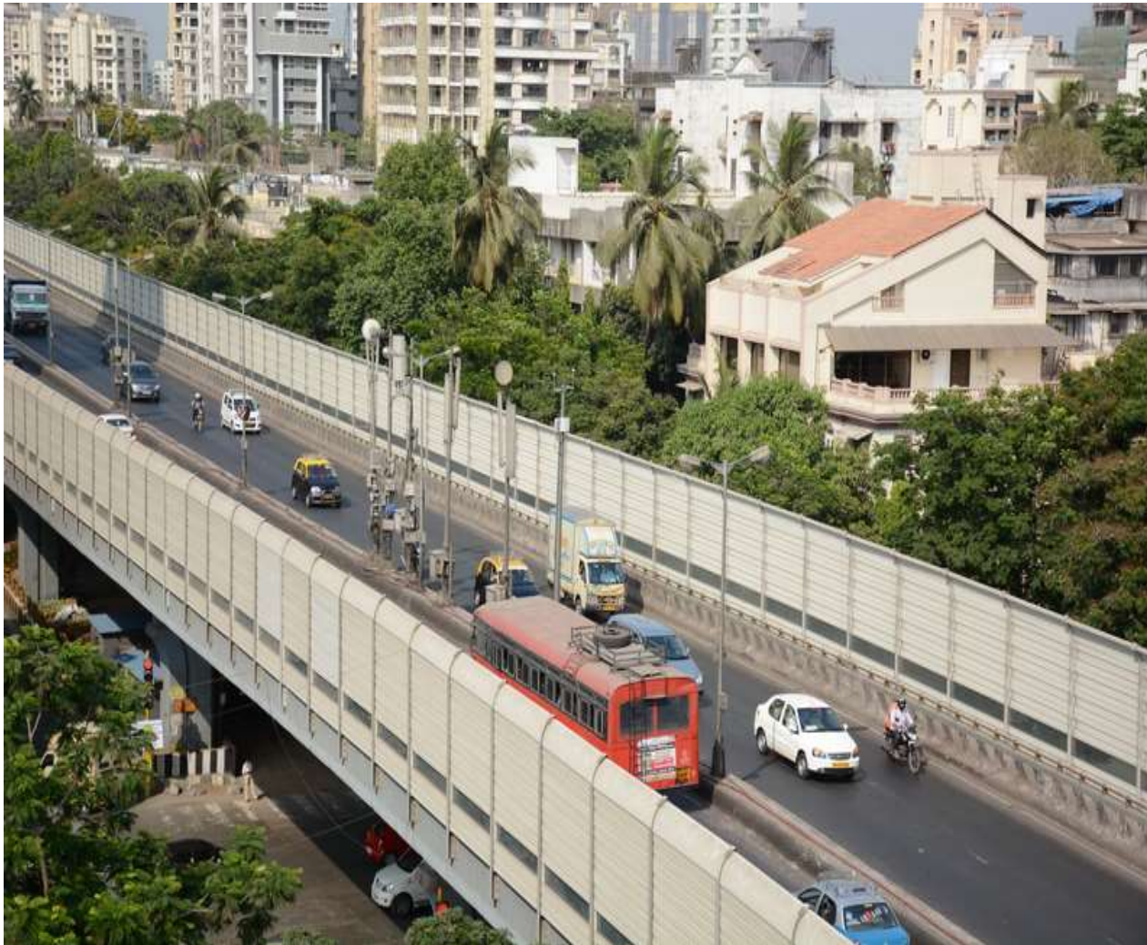
Flyover Mumbai, India
