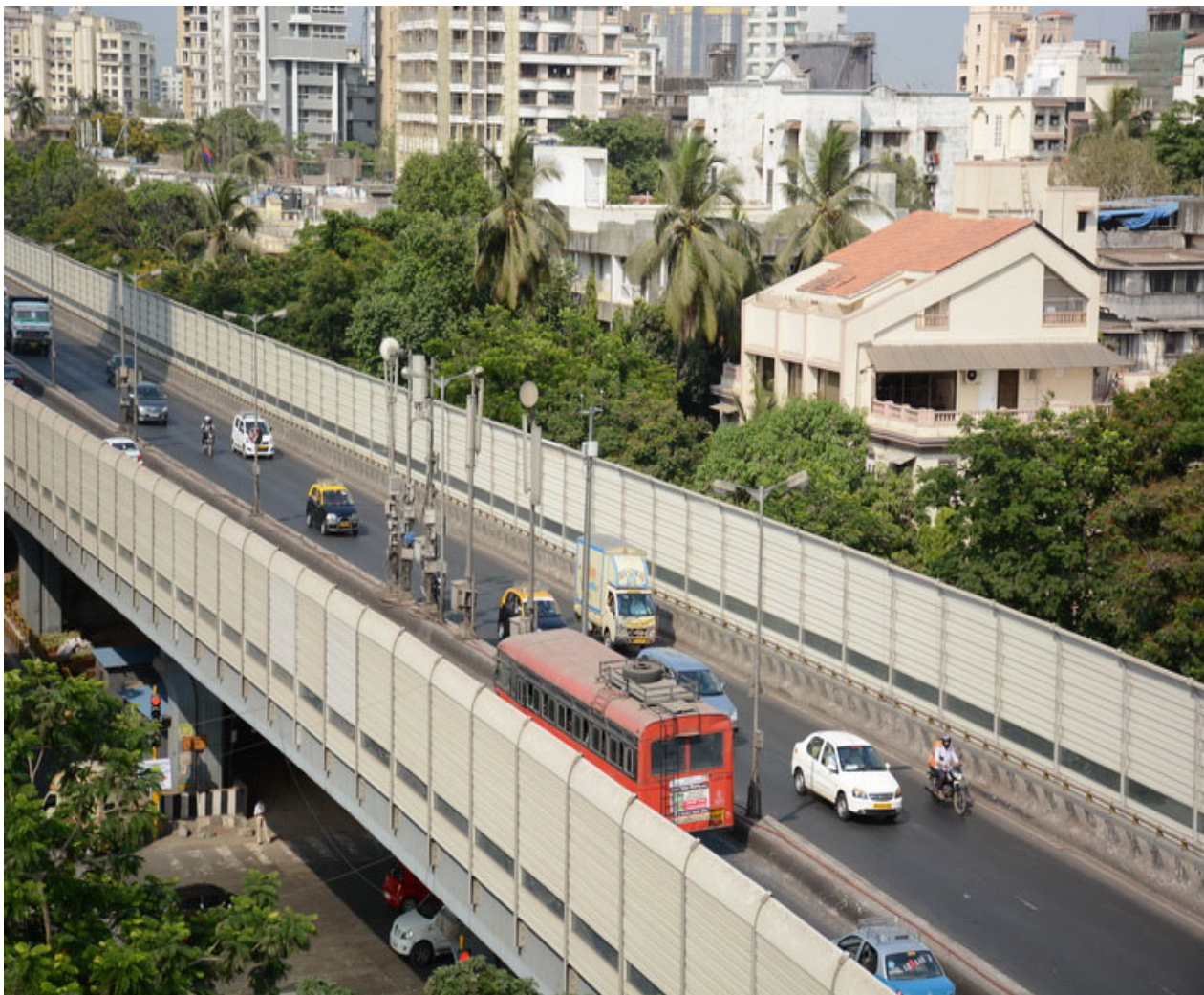
Flyover Mumbai, India
